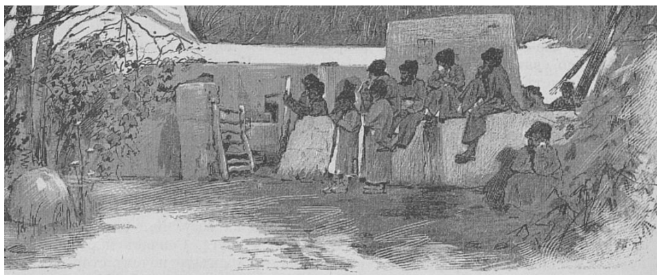
Fig. 1. Clay elevations - syra , in the courtyard of the house of Yusup Khan in Merv. Drawing by V. Pavlov. In the foreground of the drawing shown a syra with a wall for shade; in the background is a night syra .
